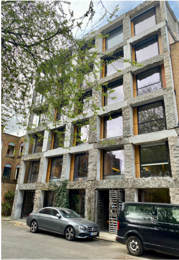
Figure 4.6: The 15 Clerkenwell Close building in London.
