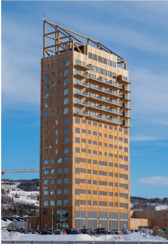
Figure 4.3: The Mjøstårnet tower at its opening in March 2019.
