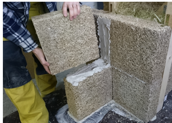
Figure 4.5: Hempcrete wall being built.
